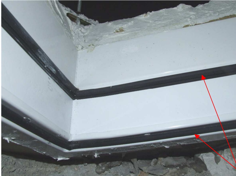
View on fixed frame of the shutter
